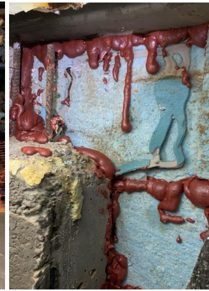
Reinspection and Manual sealing, if required
