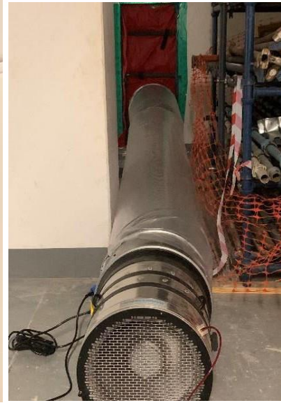
Blower door installation and Pressurization test
