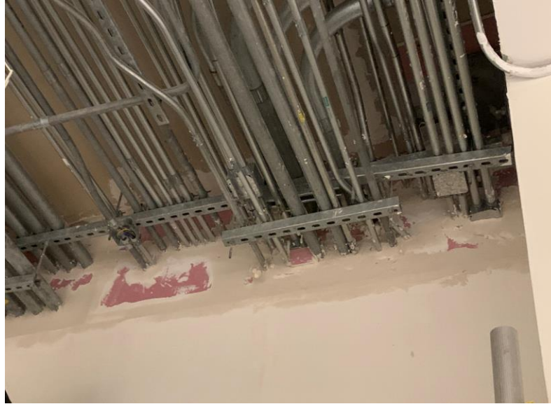
Manual sealing of large visible openings
